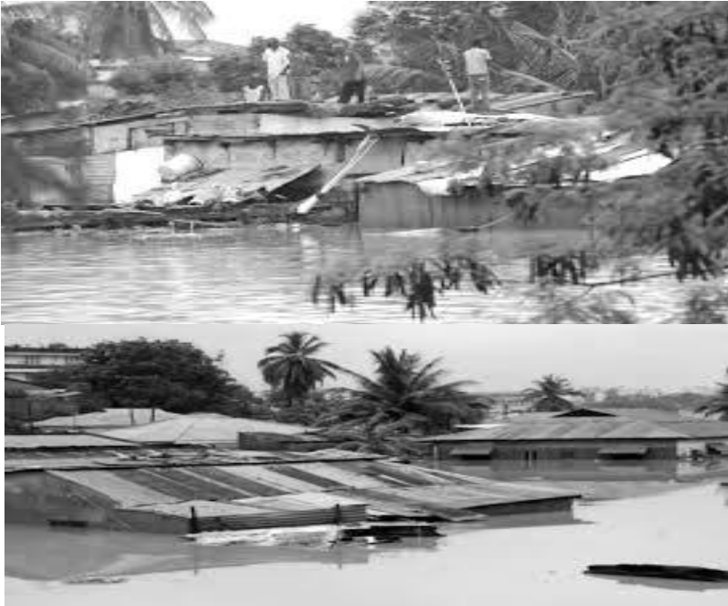
Figure 5. Floods Situation at Mtambani B February 2014
